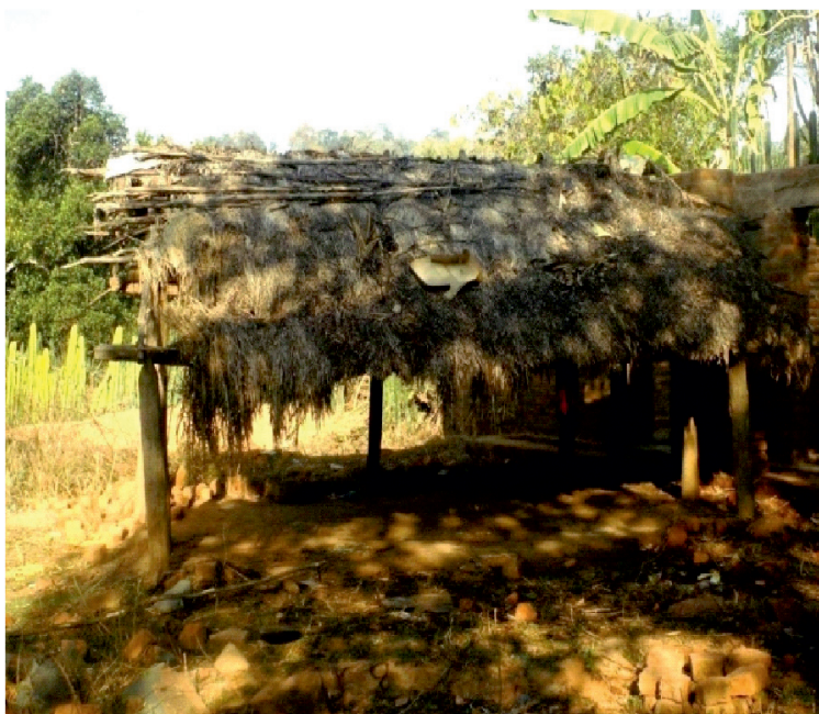
Figure 7: Reed Thatch House
